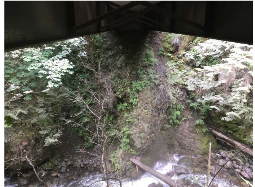
Right Bank Abutment when facing downstream
