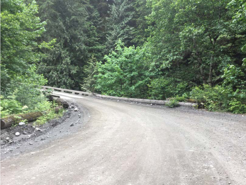
Approach from Left Bank when facing downstream
