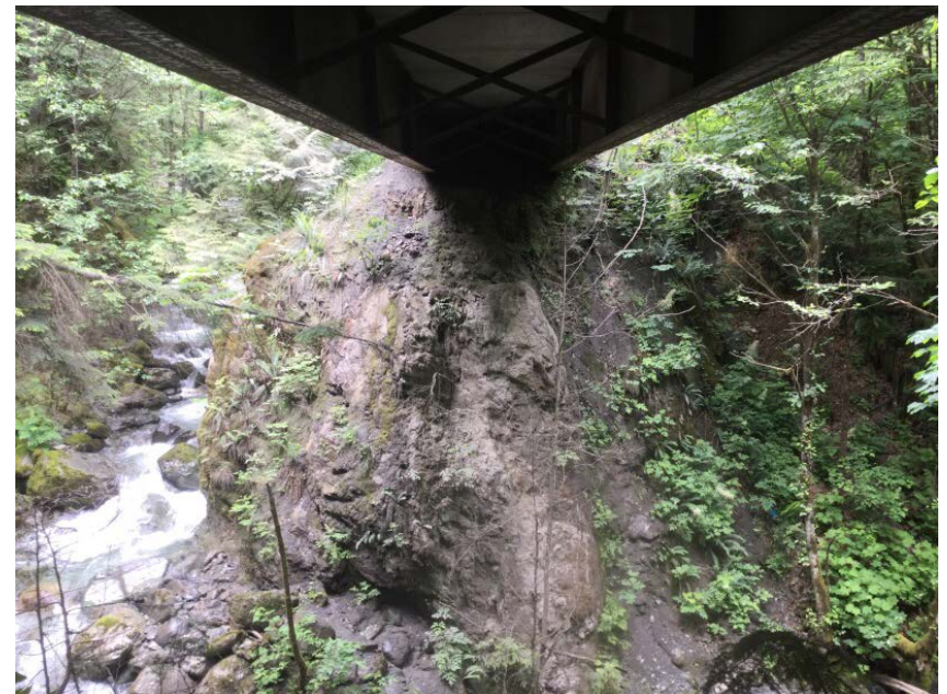
Left Bank Abutment when facing downstream
