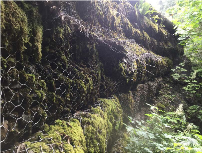
Left upstream gabion wall
